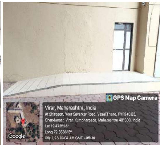
Lift and ramp
